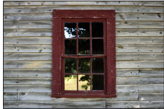
Figure 3. Barn window with wood siding. An example of a material that “looks bad before it goes bad” (source: https://pxhere.com/en/photo/569328 )
