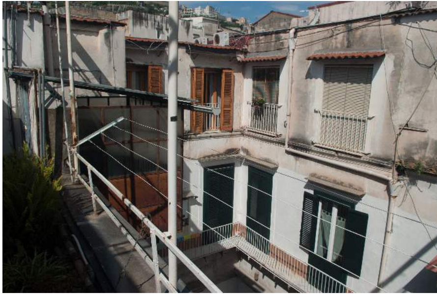
Figure 18: Additional floors and other additions on the top of a 19th century palazzo in Naples
