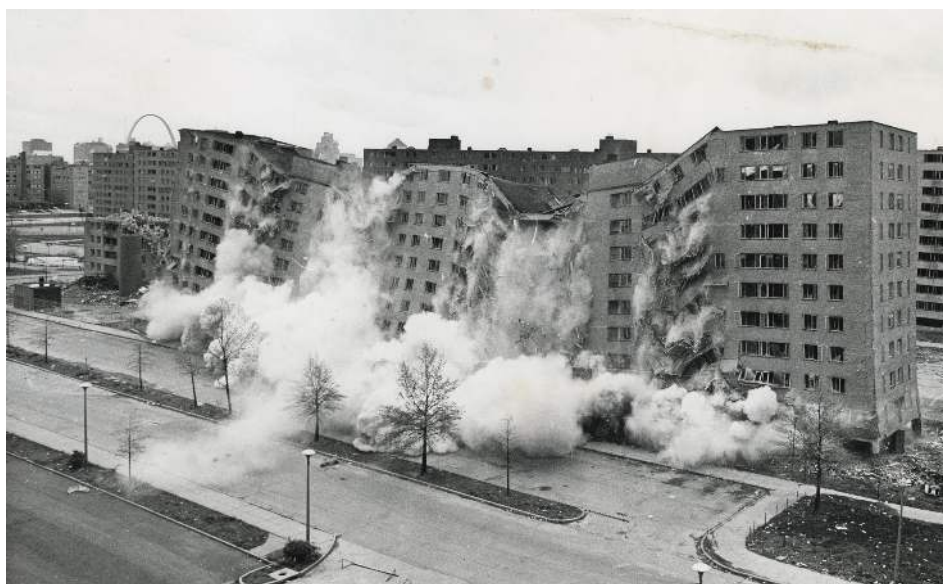
Figure 16: The demolition of the second Pruitt-Igoe building, April 21, 1972.
